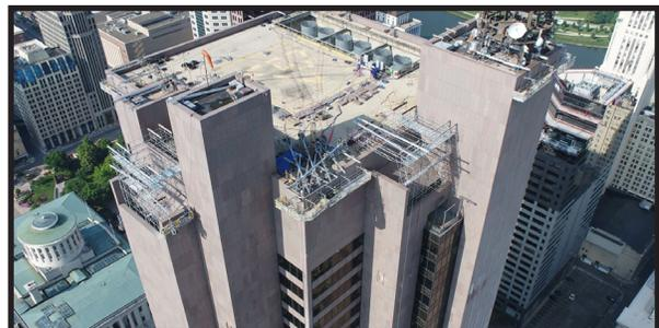
Drone-captured photos show the roof of the Rhodes Tower and the northeast side of the building. The northeast side is the elevation where the window-replacement project will begin.
